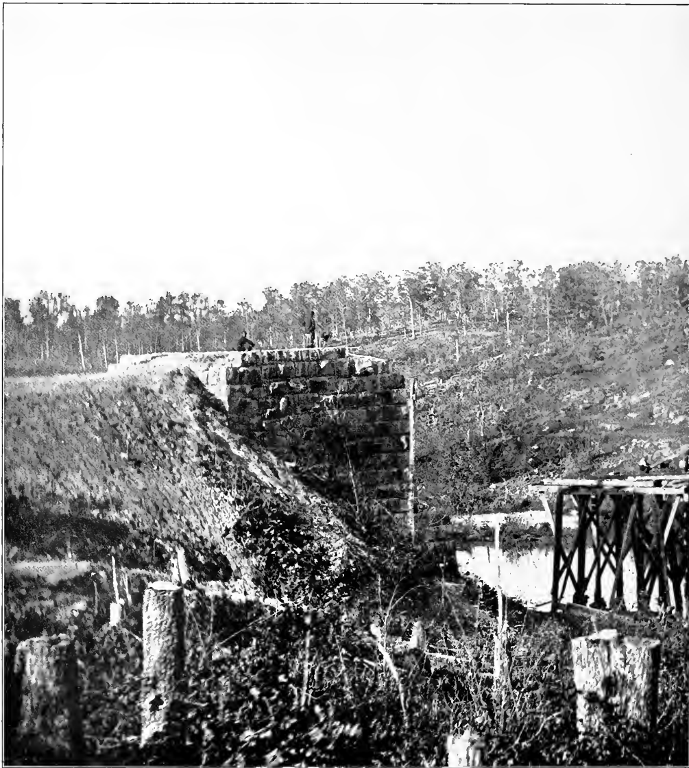
REPAIRING CONFEDERATE DAMAGE
